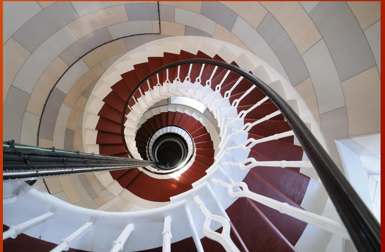
Spiral staircase inside the Isle of May Lighthouse, Fife, Scotland
